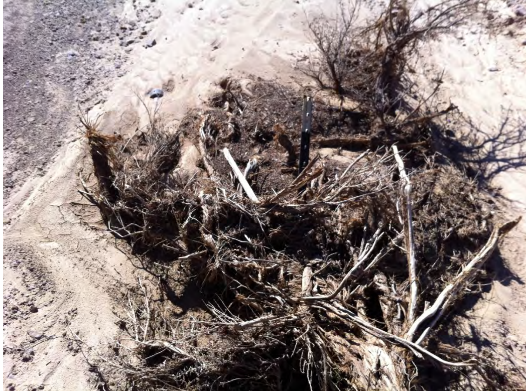
Photo of one of the more severe events – Note the bent T-post and buried Crest Gauge
