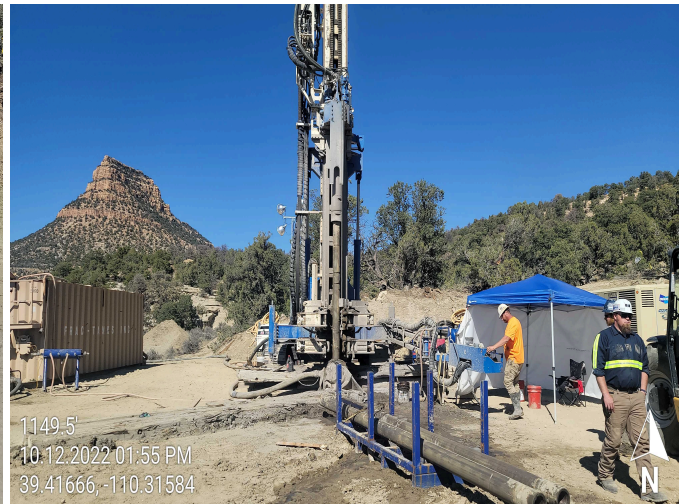
Photo 10 Borehole #2 had just broke through to the crosscut, 1149.5 feet
