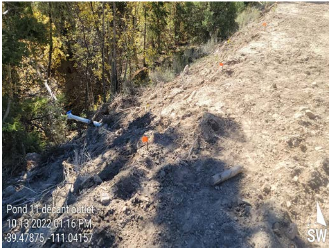
Photo 7 Pond 11 decant outlet
