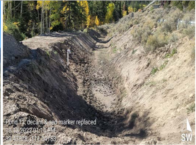
Photo 2 Pond 11, decant and sediment marker replaced
