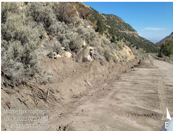
Photo 11 Middle fork road repair (2)
