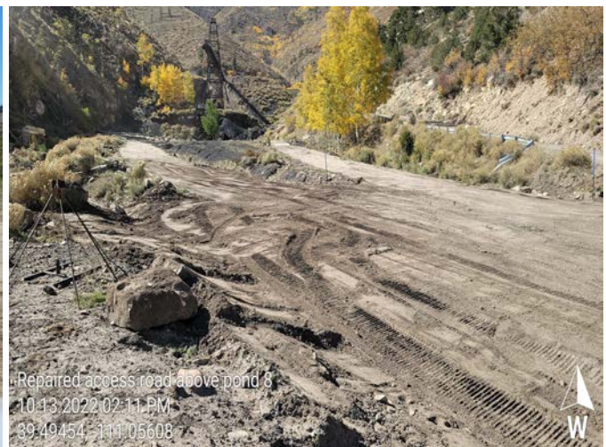
Photo 12 Repaired access road above pond 8
