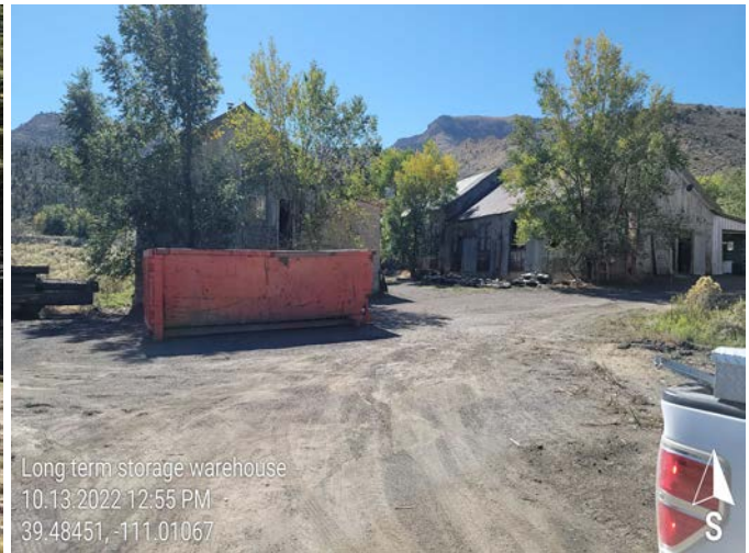
Photo 4 Long term storage warehouse
