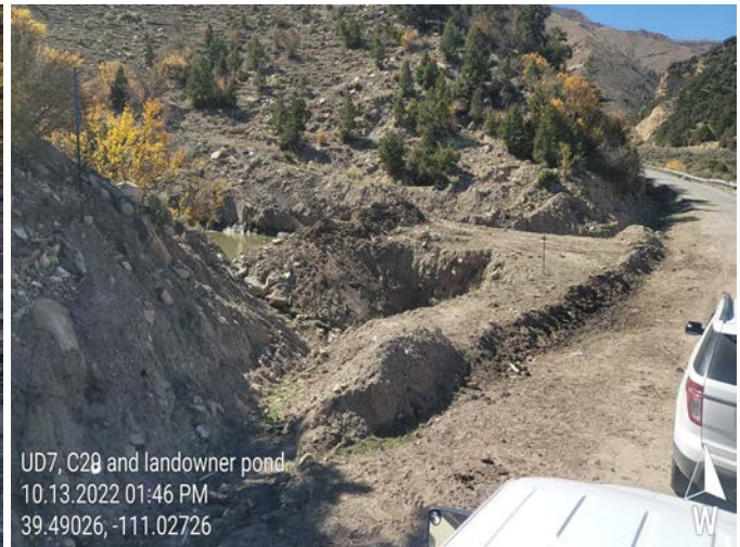
Photo 10 UD7, C28 and landowner pond
